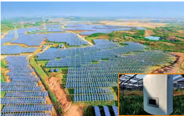
Zhejiang Hangbu Agricultural-photovoltaic hybrid PV plant 30MW
