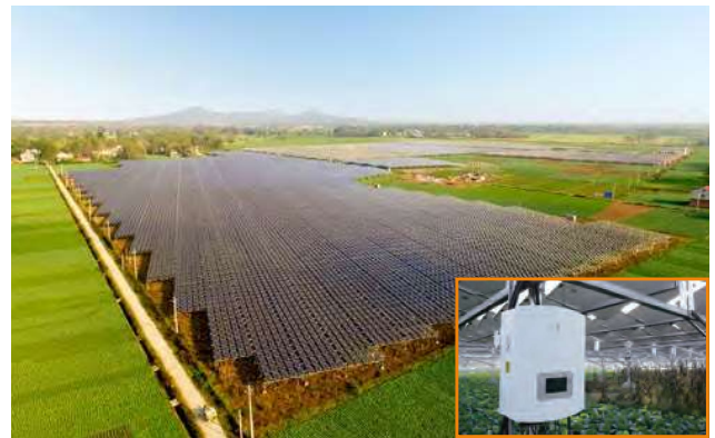
Hubei Guanyin Agricultural-photovoltaic hybrid PV plant 20MW
