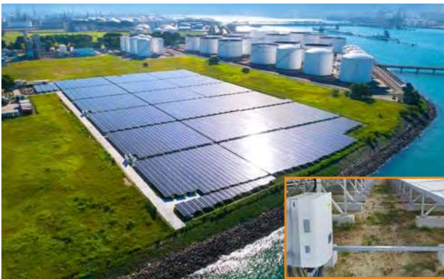
JTC Solar Farm, Singapore 5MW
